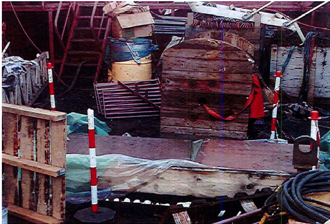
Figure 5: The state of the main deck after the incident: timber and metal sheets cover the maintenance hatch, and four red and white posts have been put up as a precaution. The area around the maintenance hatch is obstructed by building materials.
