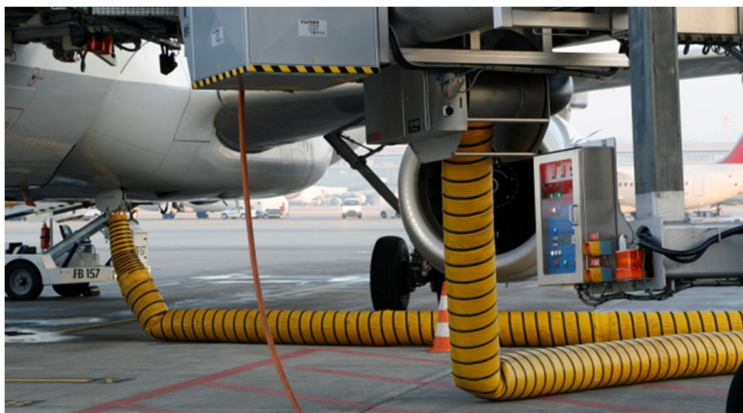
Figure 5: Air hose of the pre-conditioned air system connected to the low pressure ground connectors. Source: Zurich Airport.
