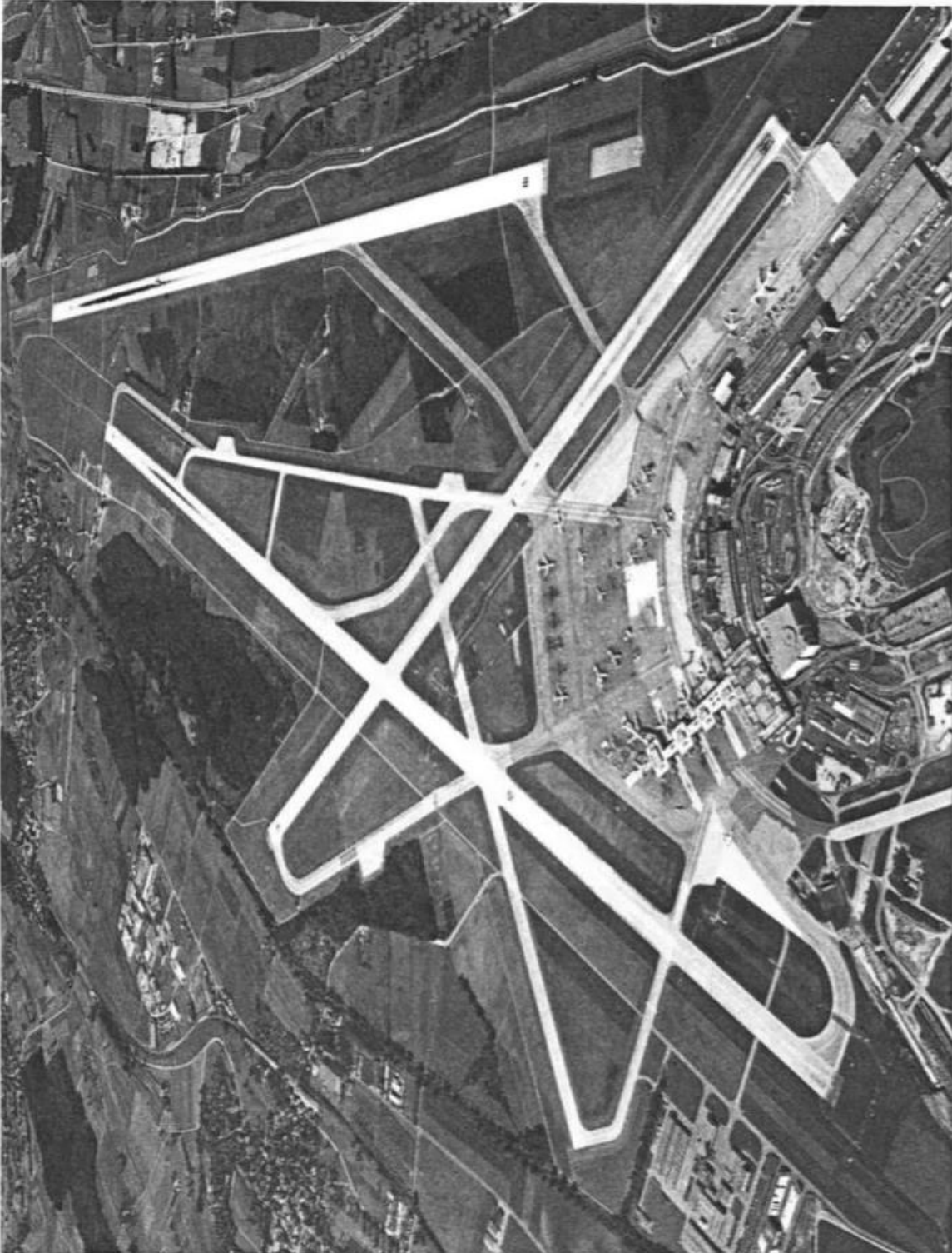
AERIAL VIEW OF ZURICH AIRPORT LAYOUT.
