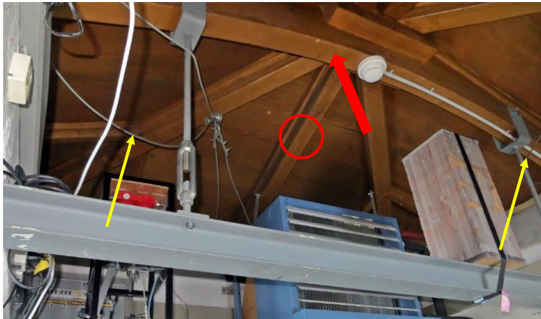
Figure 6: Interior view of the roof. The thick red arrow indicates the main beam. The red circle marks one of the two roof rafters. The yellow arrows indicate the two pre-mounted wire rope slings in the main beam.
