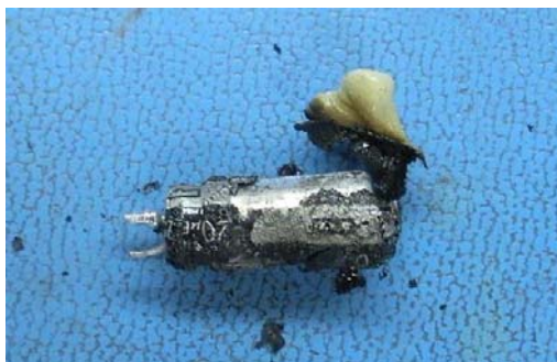
Fig. 6: Capacitor C12 overheated
