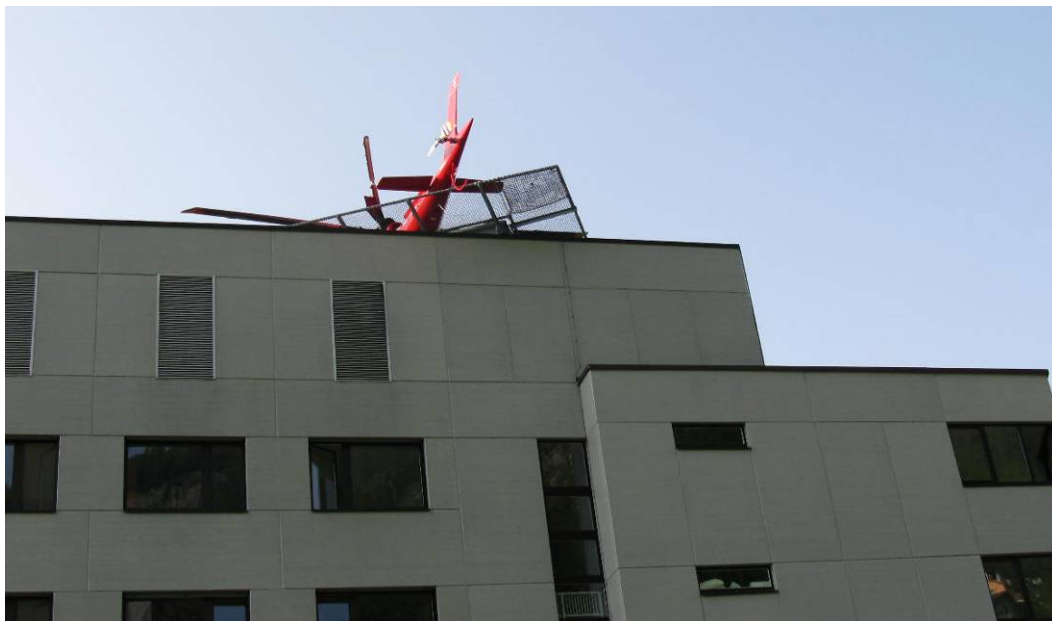
Figure 1: The damaged helicopter extends beyond the helipad and the facade of the building.
