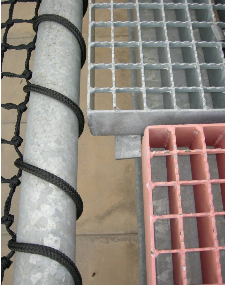
Figure 4: Displaced grating
