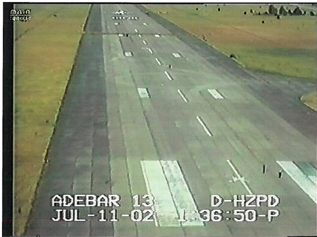
View of the runway shortly prior to over-flying the aiming point markings of the original Runway 08. In the background the earth wall, after that the runway threshold markings on the approved Runway 08, and the position of the aircraft. Film still: Police
