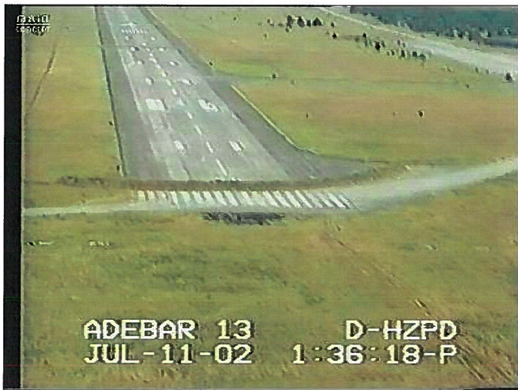
View of the new threshold to runway 08 a distance of about 1.2 km
