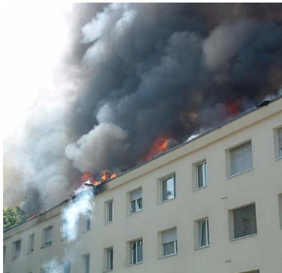
Fig. 7: Attic of the property at Roggenburgstrasse 9 – 15 on fire
