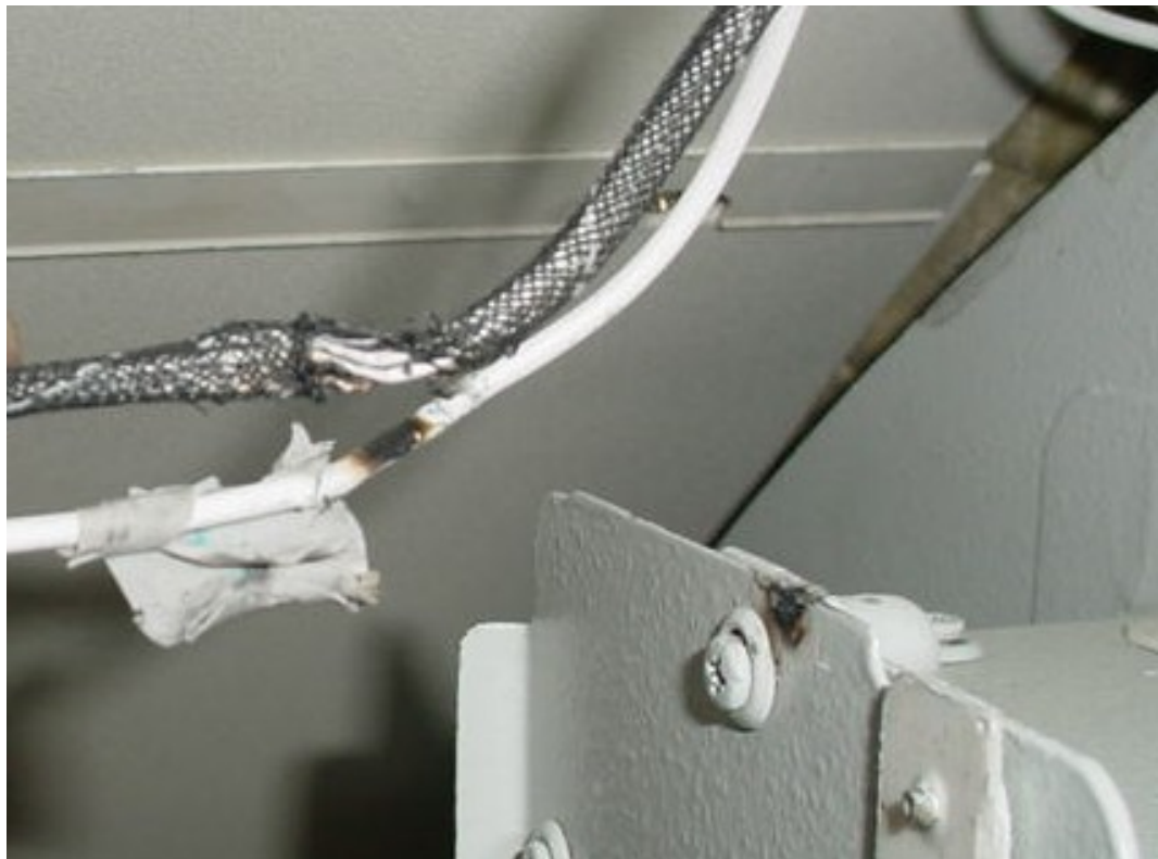
Figure 1 – Damage behind the forward galley: the insulation of the cables is damaged. The heat marks on the cables and the aircraft structure show that arcing has occurred.
