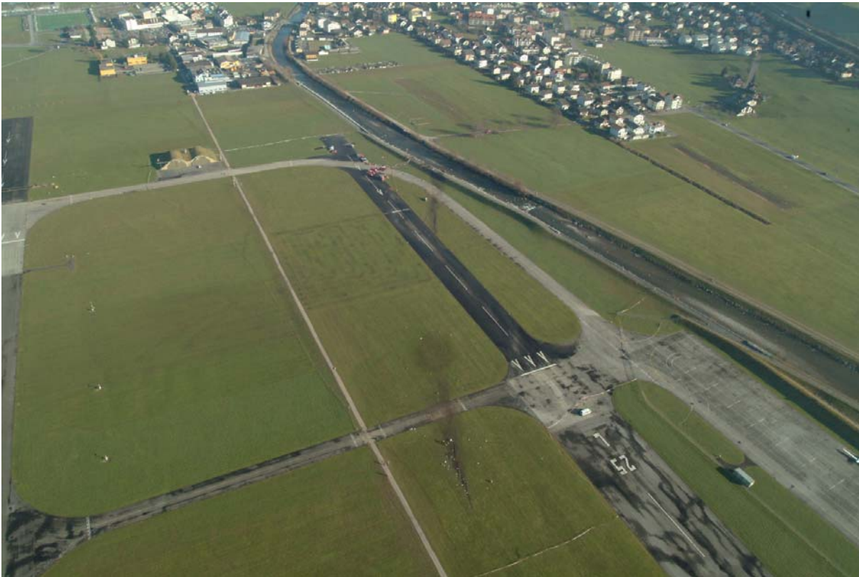
Overview in direction east
